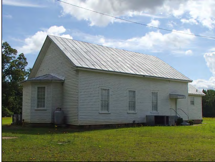
Figure 13: Autrey's Creek Primitive Baptist Church, west corner
