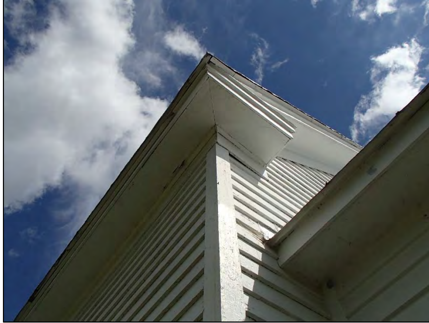
Figure 15: Autrey's Creek Primitive Baptist Church, cornerboard and eave/gable return detail
