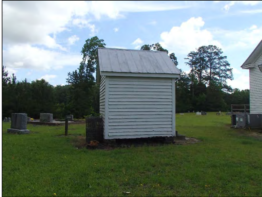
Figure 25: Autrey's Creek Primitive Baptist Church, outbuilding, southwest elevation
