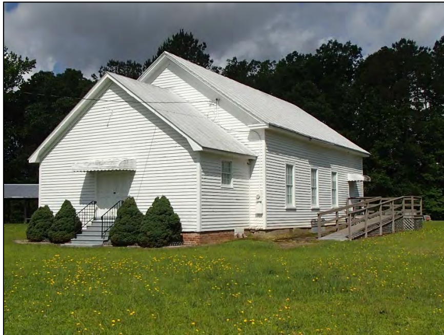
Figure 7: Autrey's Creek Primitive Baptist Church, east corner
