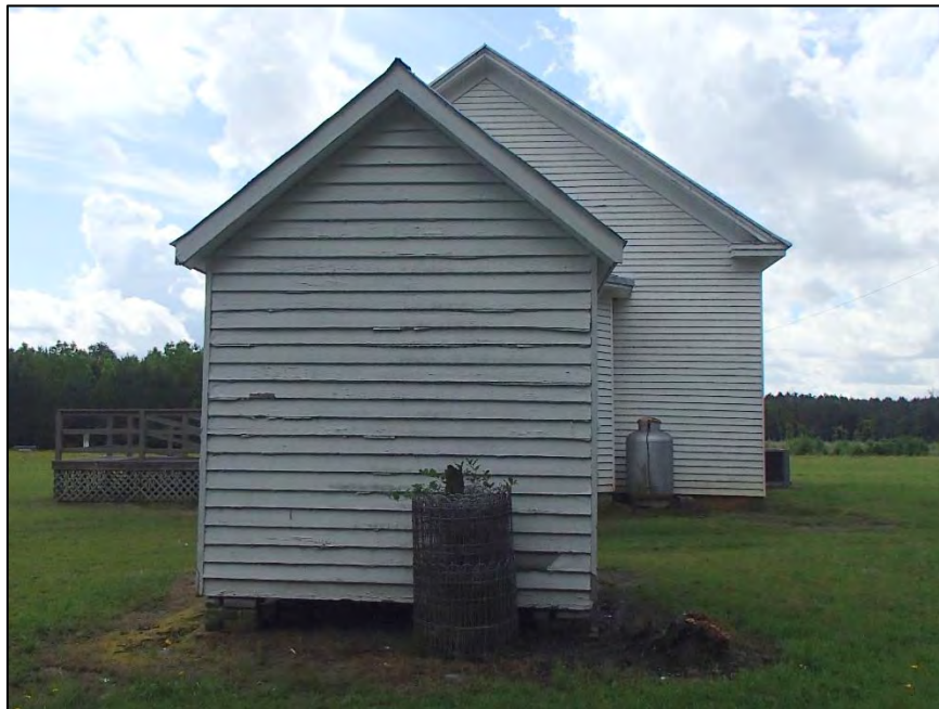
Figure 24: Autrey's Creek Primitive Baptist Church, outbuilding, northwest elevation
