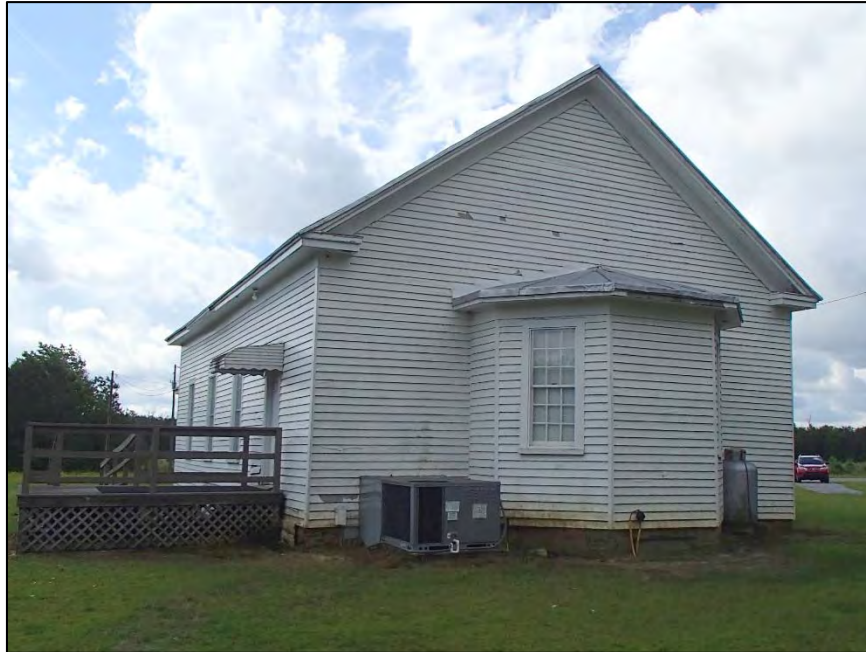
Figure 11: Autrey's Creek Primitive Baptist Church, northwest elevation
