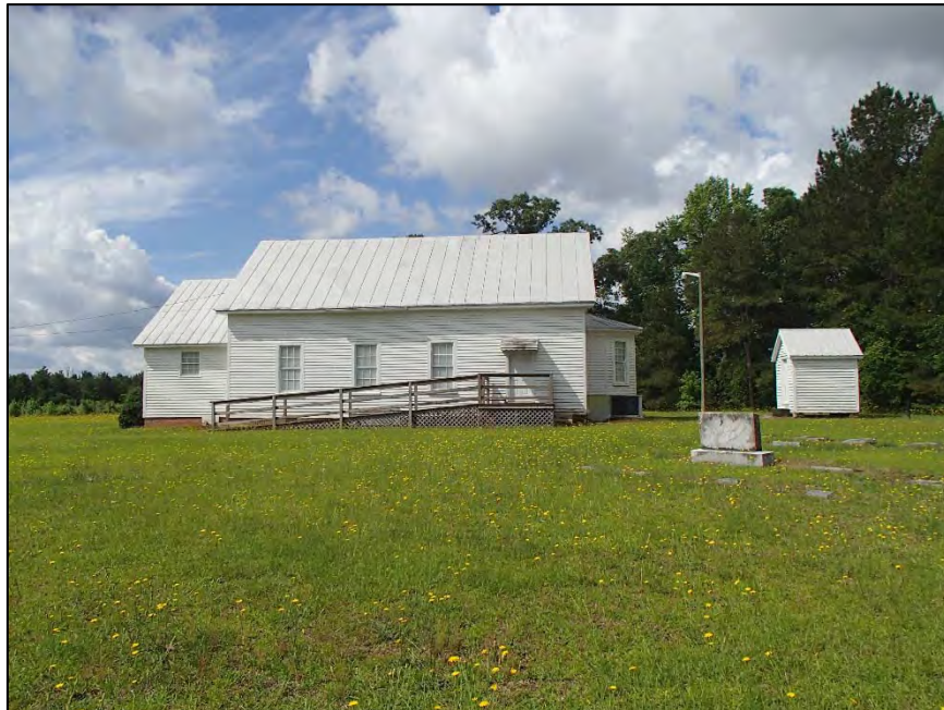
Figure 9: Autrey's Creek Primitive Baptist Church, northeast elevation
