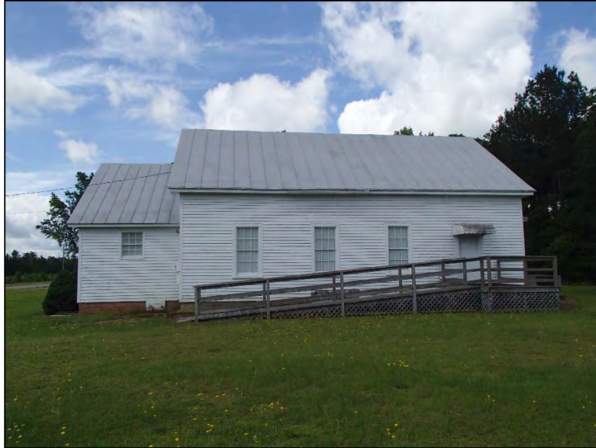
Figure 8: Autrey's Creek Primitive Baptist Church, northeast elevation
